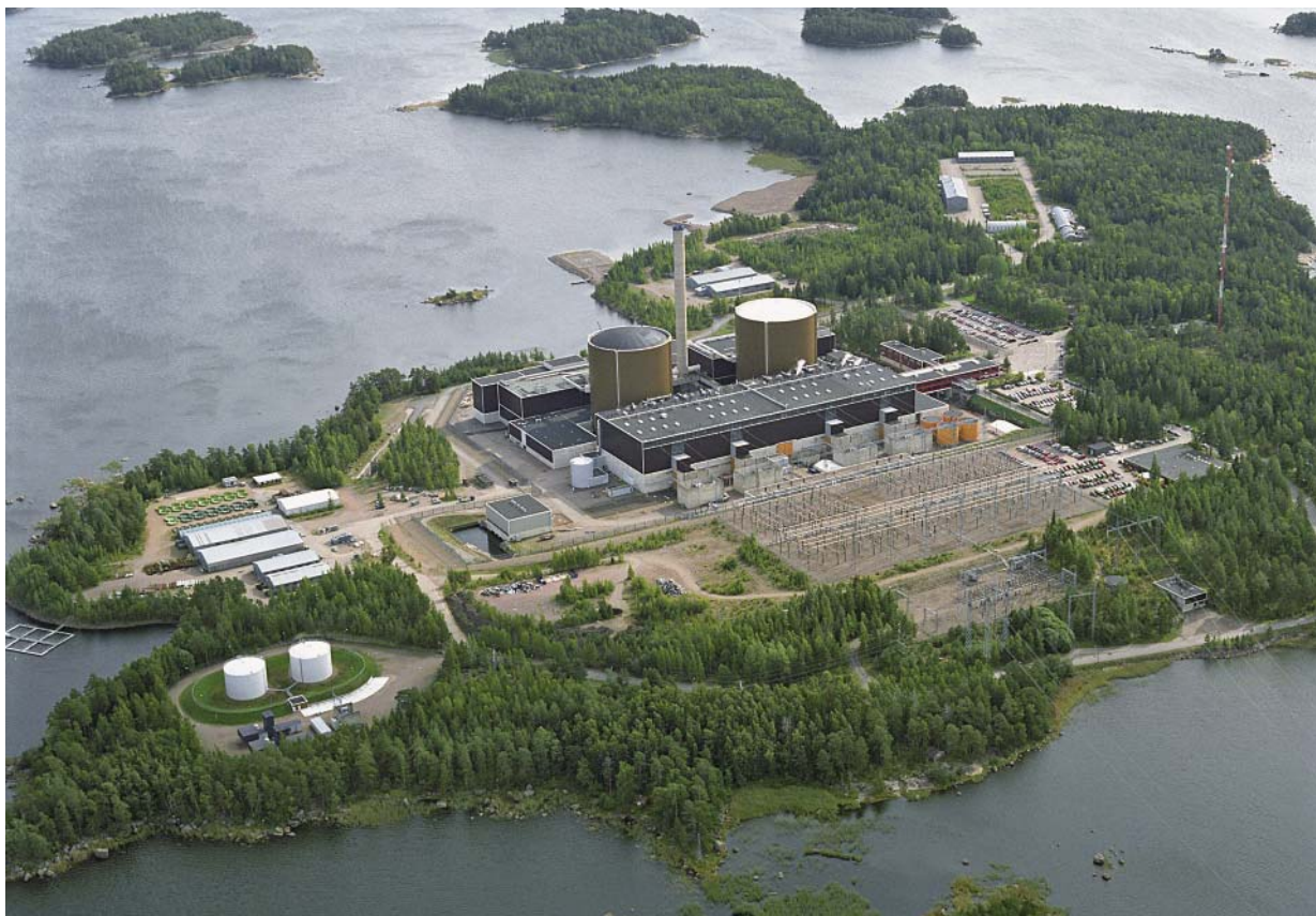
Figure 6-5. An aerial photo of the plant and its surroundings.
