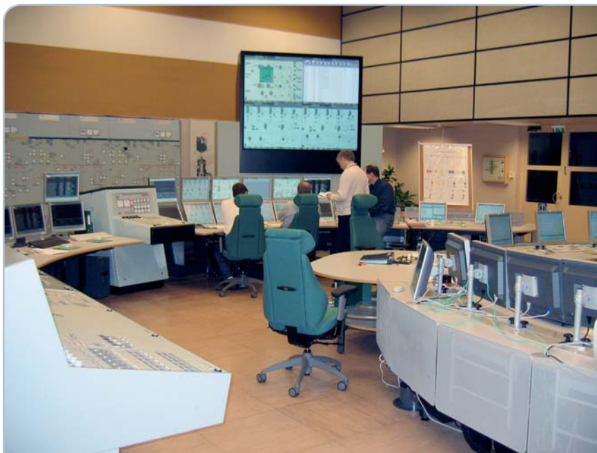
Figure 3–5 Control room of the training simulator for OL1 and OL2 plant units.
