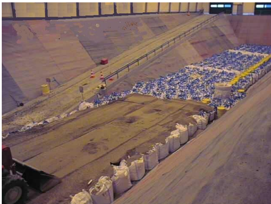
Fig. C-IX. 7 Backfilling of covering layer of soil on the first VLLW layer at repository in Morvilliers [L-110]
