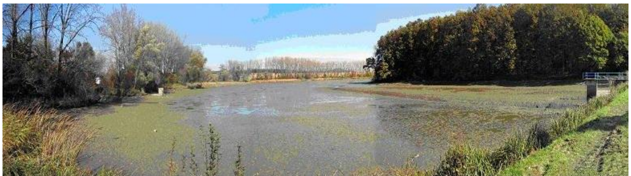
Fig. C-IX. 14 Reservoir Čifáre (Čifársky pond) with discharged water
