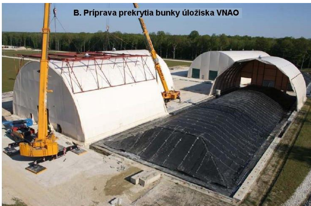
Fig. C-IX. 5 An example of VLLW disposal at Morvilliers in France [L-110]
