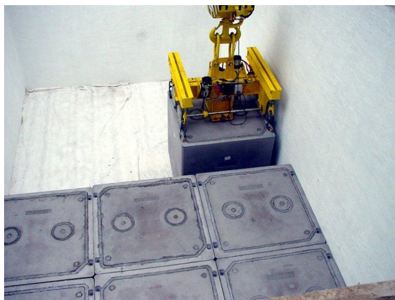
Fig. A-II. 9 Disposal of FCC in the boxes [L-66]
