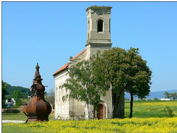
a) prior to reconstruction
