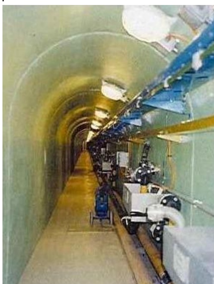
Fig. A-II. 5 Monitoring gallery of NRR Mochovce with the system of controlled drainage KD1 and KD2
