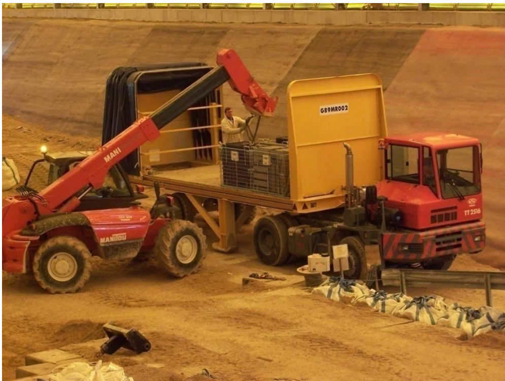
Fig. C-IX. 6 Handling with VLLW package forms at repository in Morvilliers [L-110]
