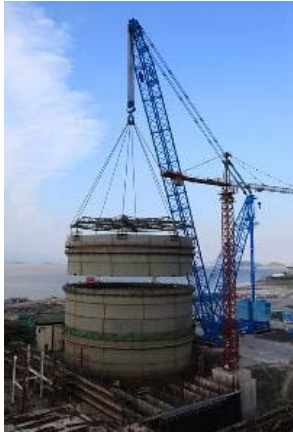
Figure 2.4.4.1-1. Placing the third containment ring at the site of Sanmen 1
