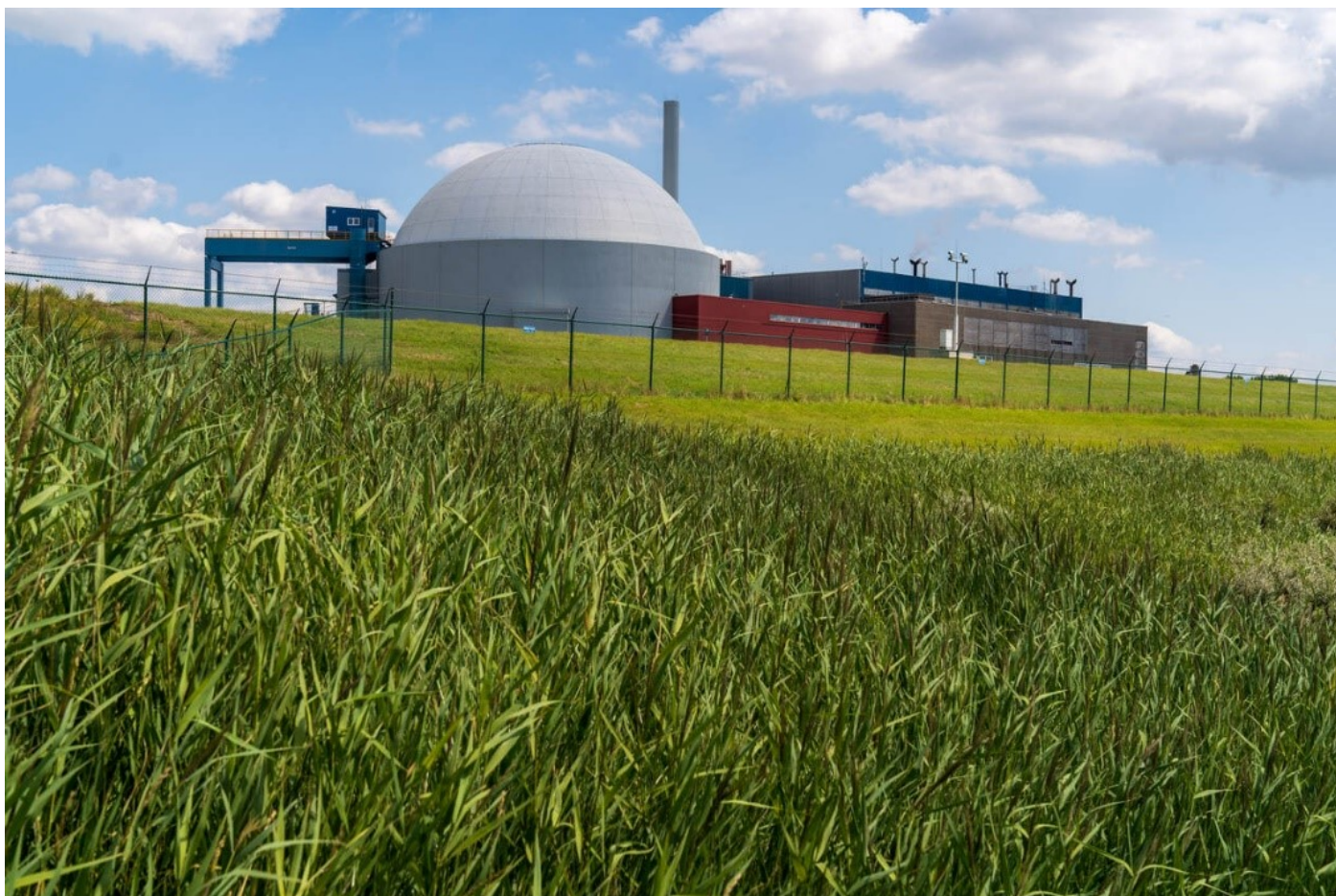
Figure 2 Borssele nuclear power plant
